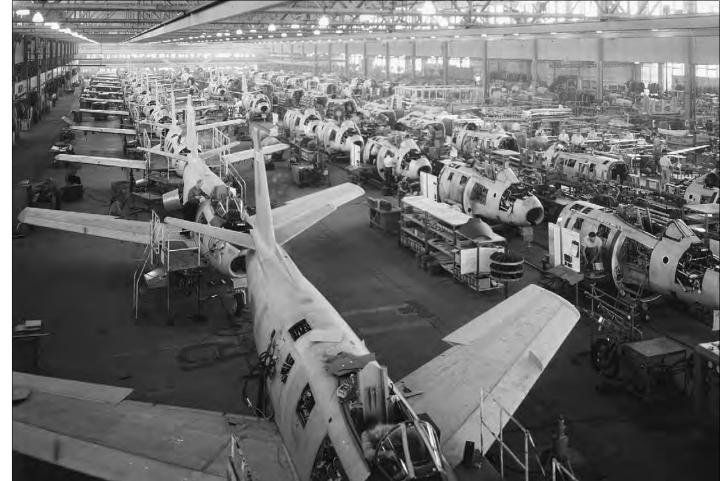
The assembly line in Montreal that produced the Canadair Sabre F-86. More than 1,800 of the jet fighters were built from 1950 to 1958.
